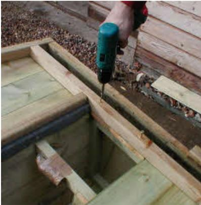
Finally screw the nest box to the frame with the screws provided through the two pre drilled holes on both sides. Then screw the two centre screws through the bottom frame into the nestbox partition spars
